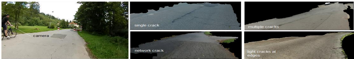
Figure 1. (Left- most) Our approach for data collection using a simple HD camera mounted on a pedelac taking scene images from front viewpoint. Rest of the images show examples of pre-processed road images that are used in our approach. Few crack-types are shown.
